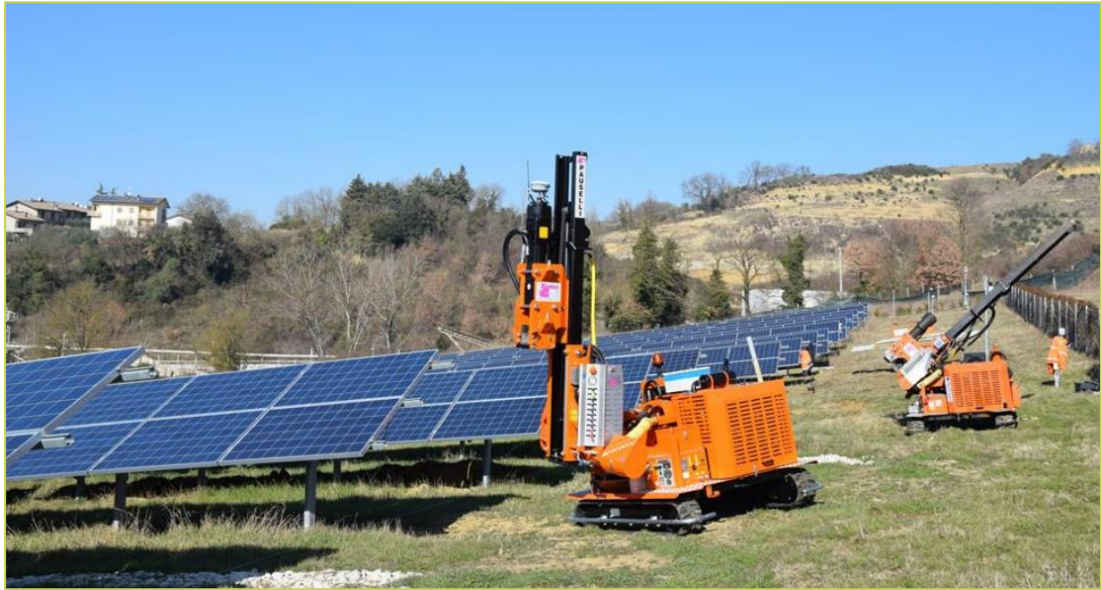
Image 4.7 Typical GPS Solar Farm Pile Driver
