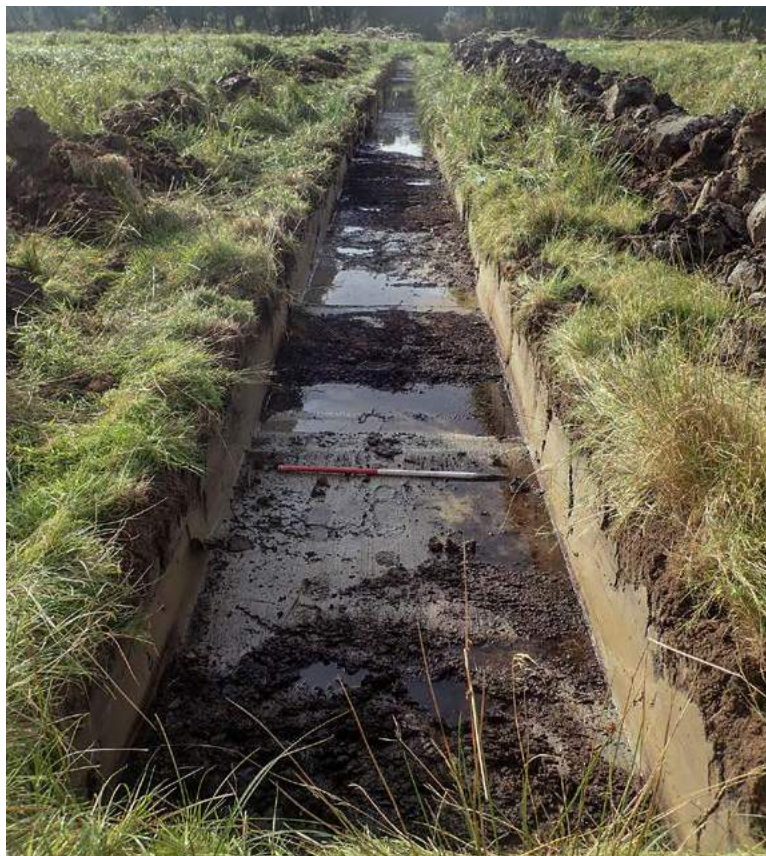
Plate 72: Area 8: Trench 123 was machined through the top part of a deep alluvial sequence, down to the surface of the peat, which was present in patches, view east, 1x1m scale
