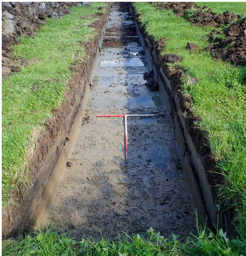
Plate 55: Area 8: Trench 111, top part of deep alluvial sequence, machined down the surface of the peat, which was only present in patches, view west, 1x1m scale
