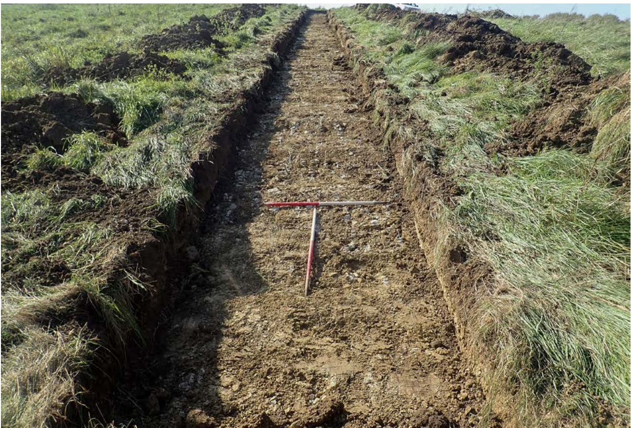
Plate 13: Area 2: Trench 30, example empty trench, view west, 1x1m scale
