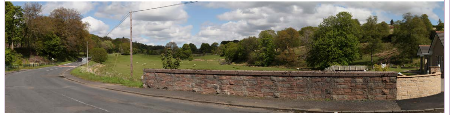
Photograph Dated: 3rd June 2015
