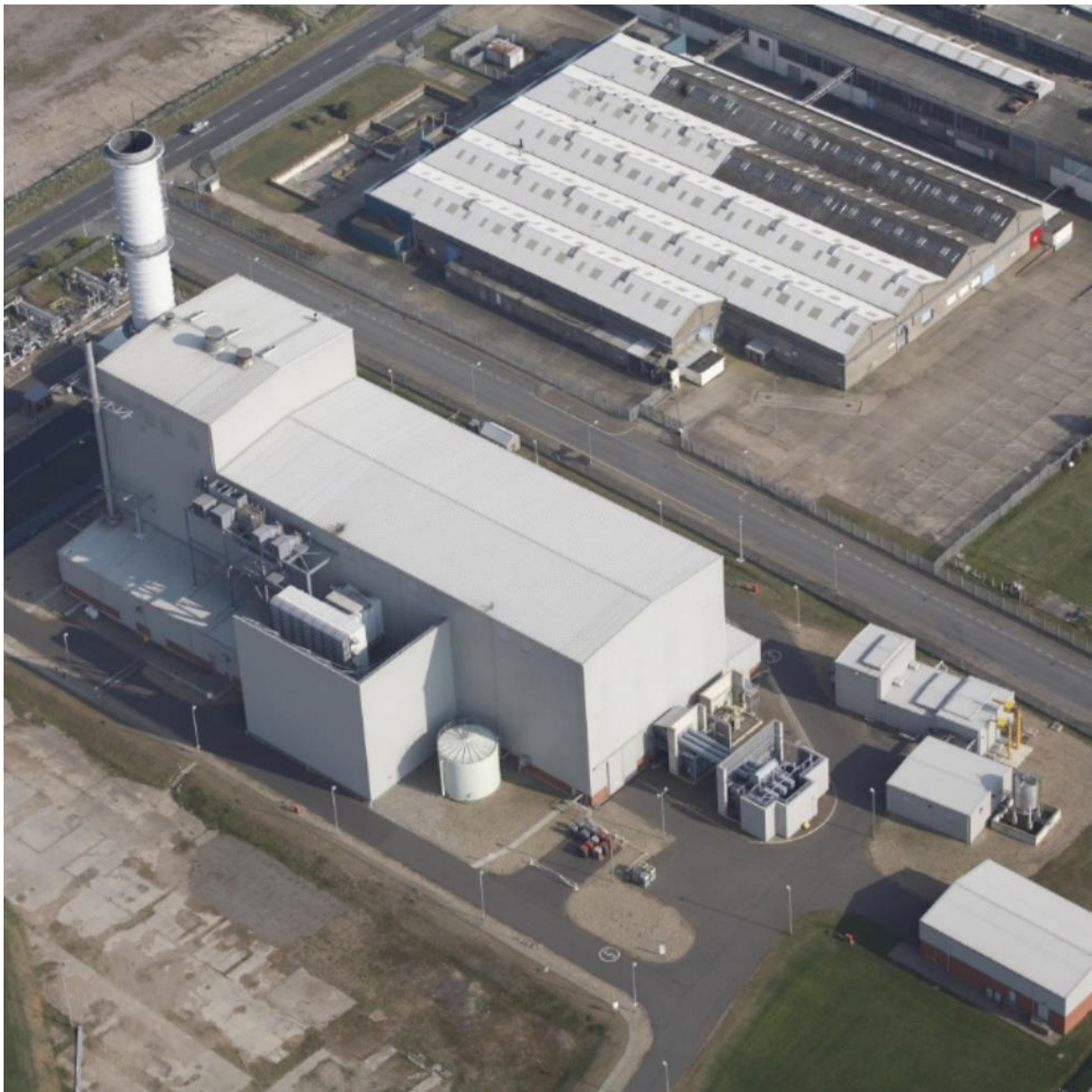
Figure 3 Aerial photograph of Great Yarmouth power station.
