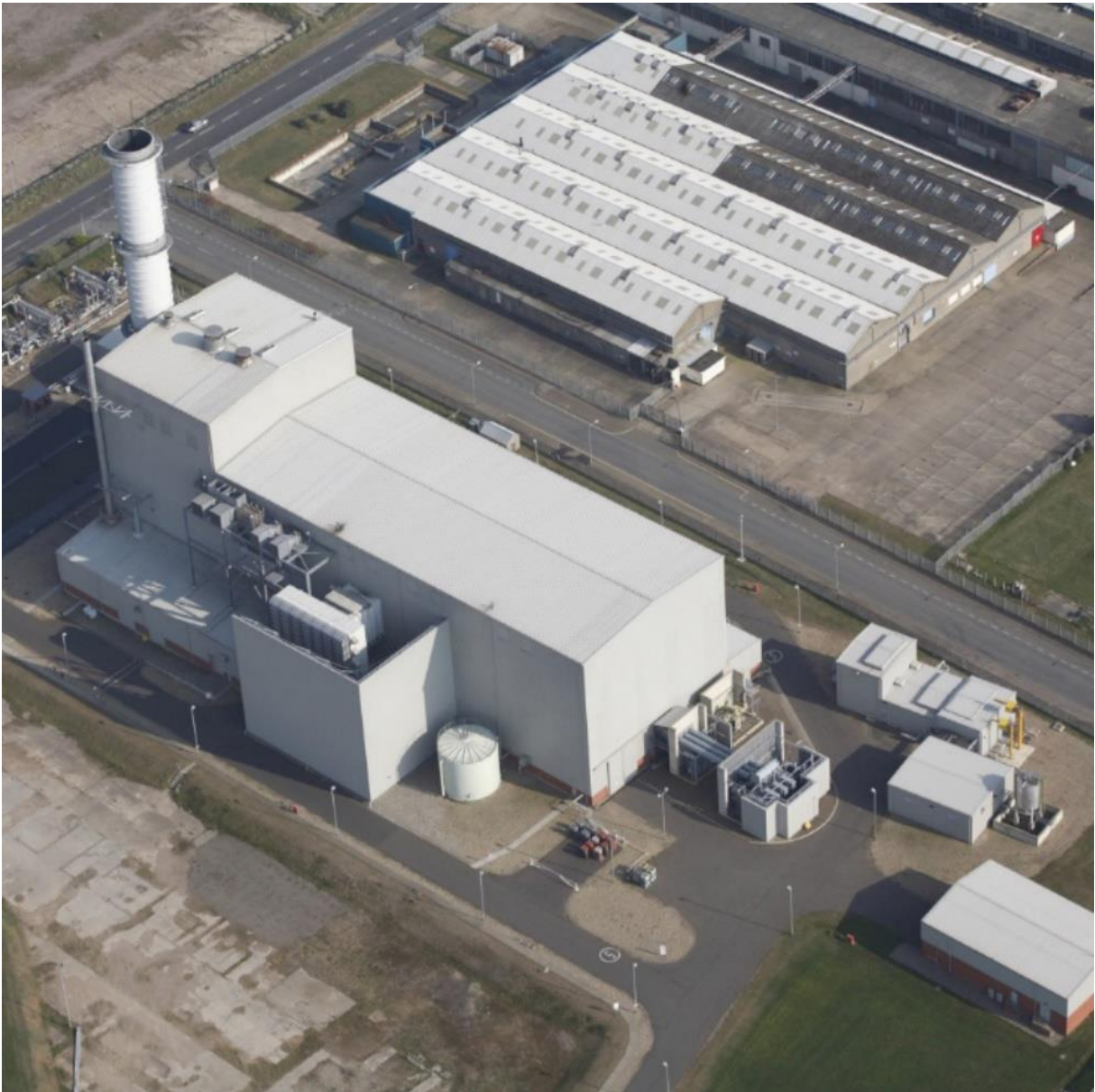
Figure 3 Aerial photograph of Great Yarmouth Power Station.
