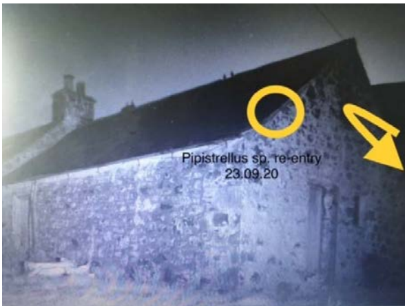
Photo 3: Re-entry point under slates at gable end of building facing southeast.
